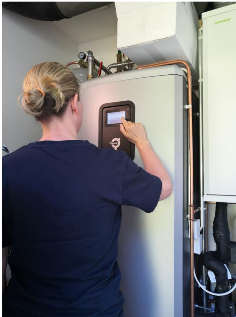
Indoor unit of a heat pump. © ELY Centre for South Ostrobothnia
