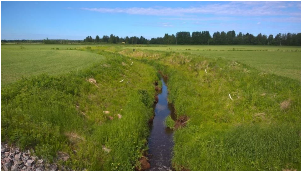
Figure 5 (Elsi Kauppinen). Two-stage drainage channel at Leppioja, a few years after construction work. Connections to subsurface drains for easier flushing are visible on the sides.
